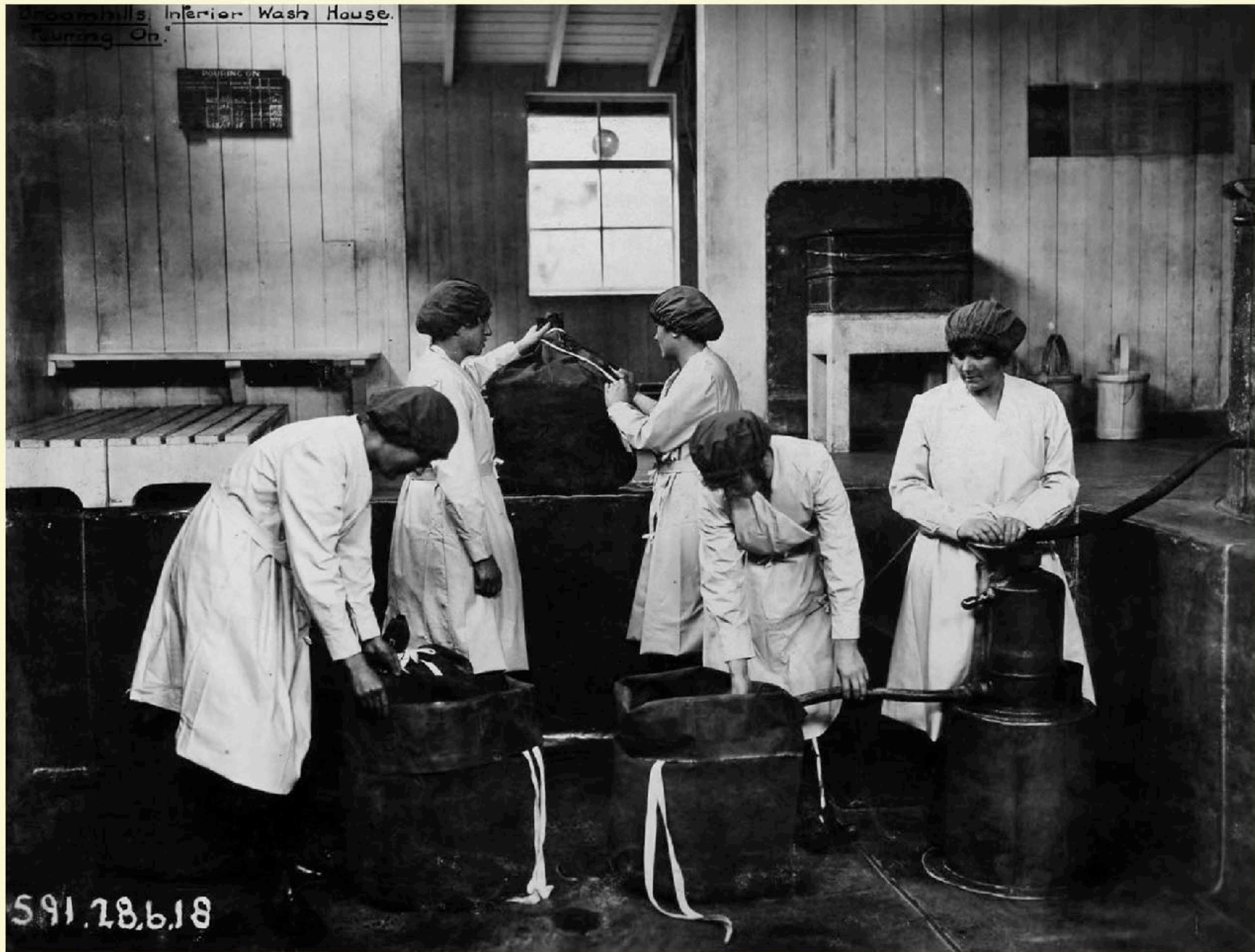
H M Explosives Factory Gretna Dumfries Wash House (catalogue reference: MUN
